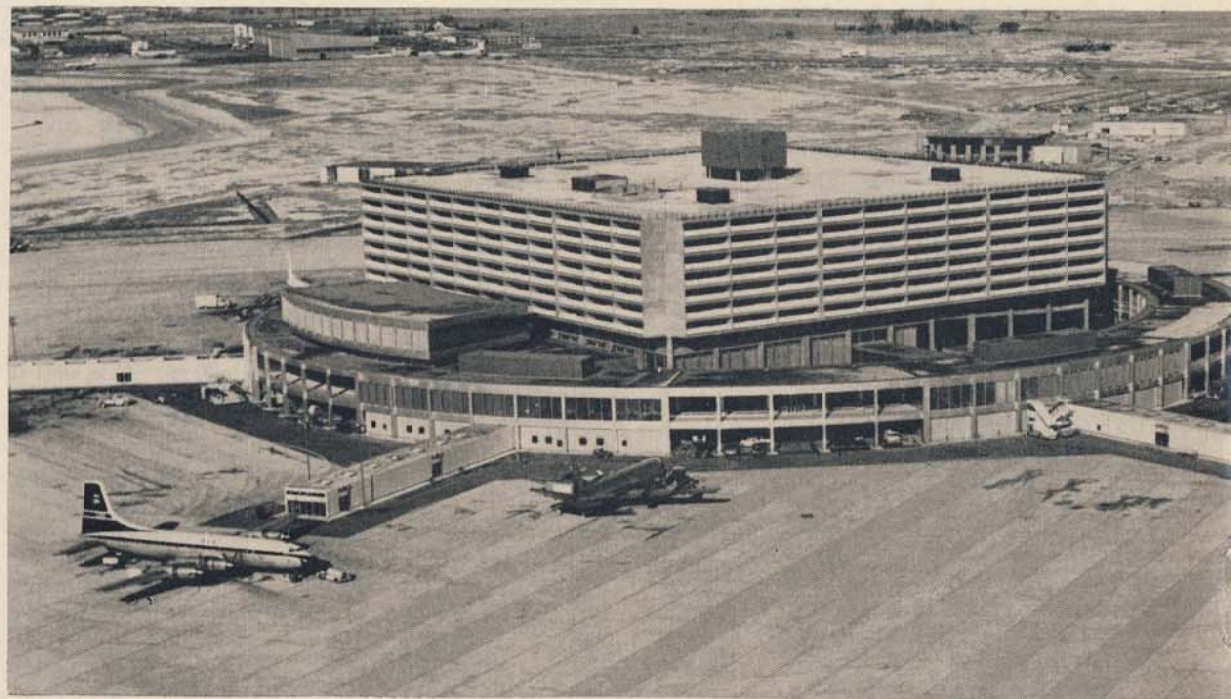
SIX FINGERS project from Toronto International Airport's aeroquay which permits passengers to walk undercover to within yards of boarding aircraft. The terminal proper on the first two floors and the eight-storey,
