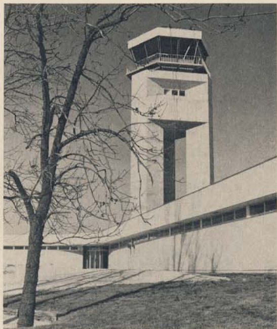
THE THREE-LEGGED control tower rises 100 feet above the air traffic control building. All immediate airline traffic is controlled from the cab on top.
